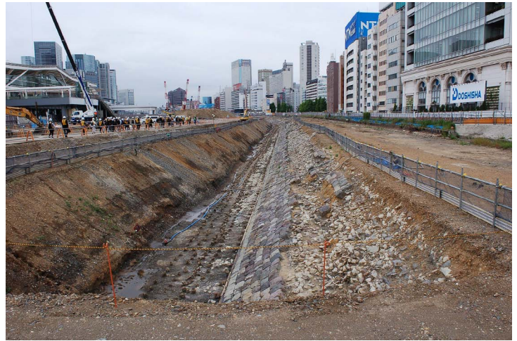
A section of the excavated Takanawa Embankment.
