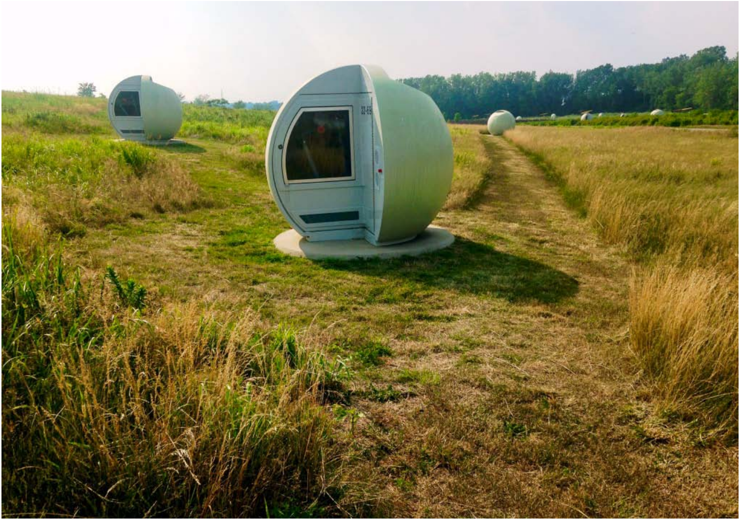
The former landfill landscape with inspection spheres revealing the biogas capture wells below.
