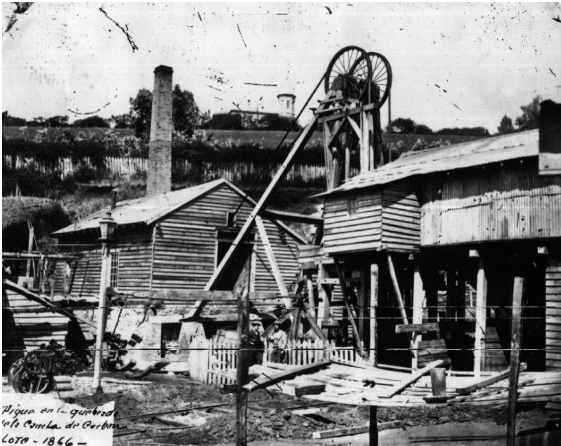
Headstock and winding engine of the mine, 1866. (ENACAR photographic record, digitized by the Universidad de Concepción Photographic Archive, recovered in 2010)
